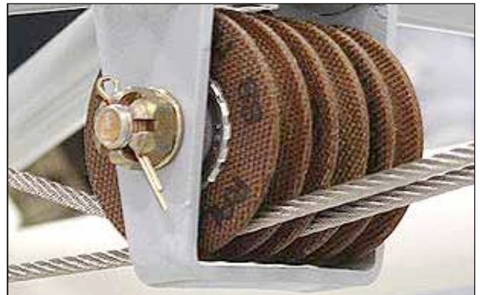
Belly control pulleys looking AFT. The far pulley, left, when looking forward is the cable from the top of the elevator bell crank. The cable from the bottom goes through the middle and the flap cable goes through the right one.
