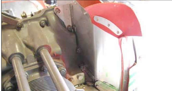
View of rear of spinner area: A nose baffle, as shown, stops circulation and leaks around the nose case/
