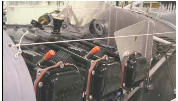
Note the relationship of the rear baffle to the string, which stretches from the nosebowl to the firewall. Van's baffles are too tall and using strings will establish the proper height.
