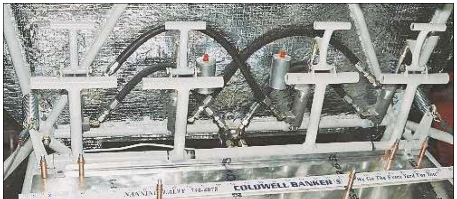
In this application the left and right master cylinders are plumbed together with the "out" lines plumbed to hard lines to the landing gear in the middle. Integral reservoirs are used on this installation.
